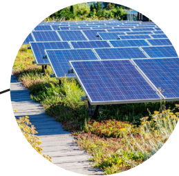
Photovoltaik + Retentionsdach
